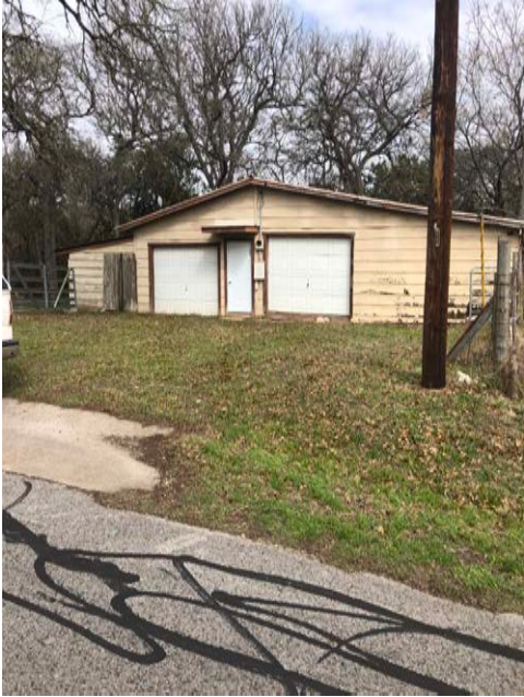
4. Front view from road
