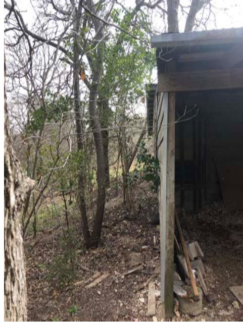
4. Back view parallel to road
